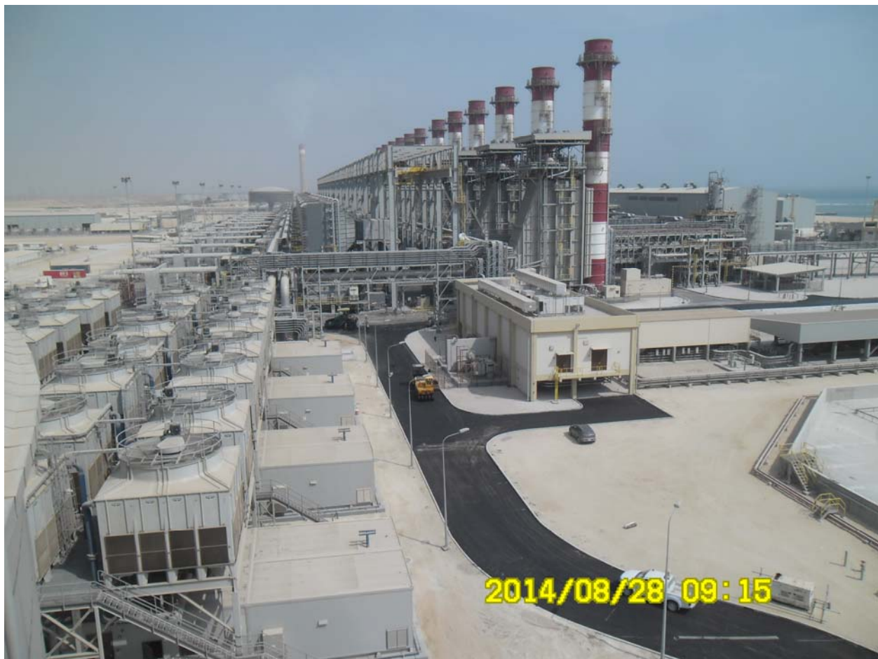
Figure 4 Power Block Overview
