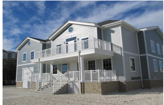
Exterior of Peerment Substation
