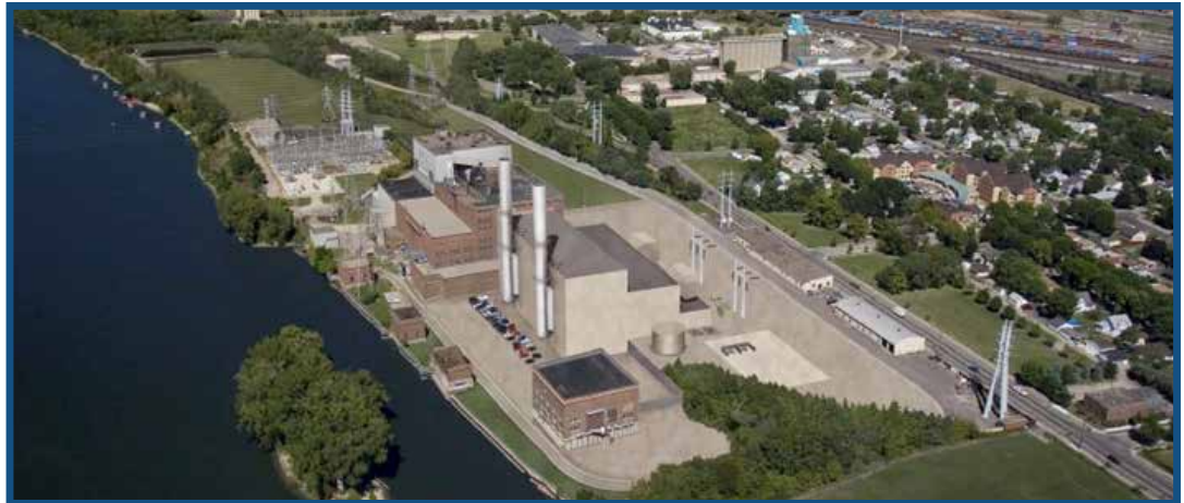
Riverside Plant, Minneapolis, MN
