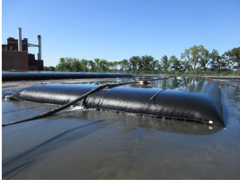
**Figure 6: A geotextile dewatering tube being filled with the CCR and sediment slurry.**
