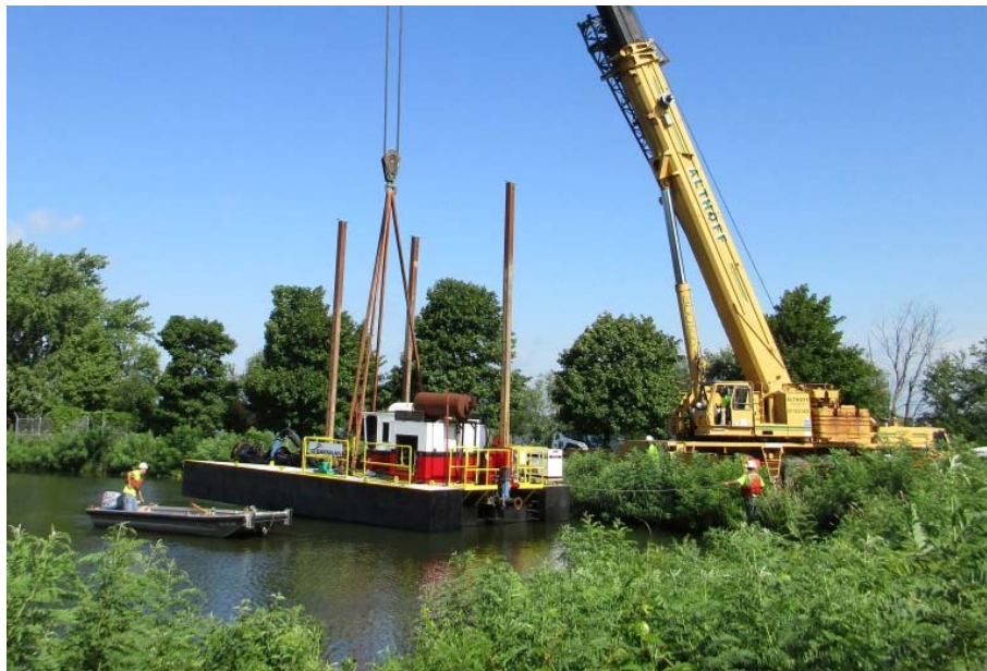
Figure 2: Deployment of the barge-mounted hydraulic dredge onto the impoundment.
