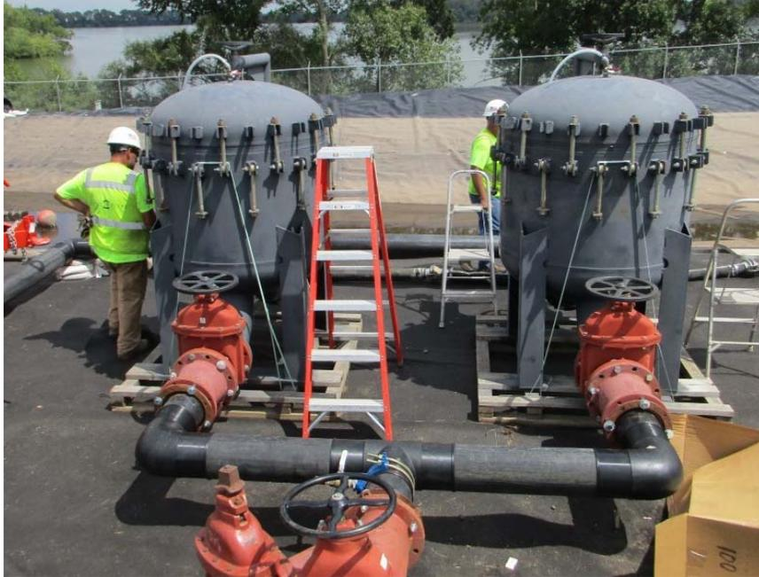
**Figure 7: The two 100-micron bag filters of the temporary water treatment plant.**
