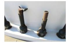
**Anchor Bolt Maintenance:** Anchor bolt tensioning procedures should be in place to periodically confirm that the anchor bolts are tensioned in accordance with the foundation design technical specifications. Procedures should indicate an interval for inspection and provide a means for technicians to classify and remediate any anchor bolt corrosion.
